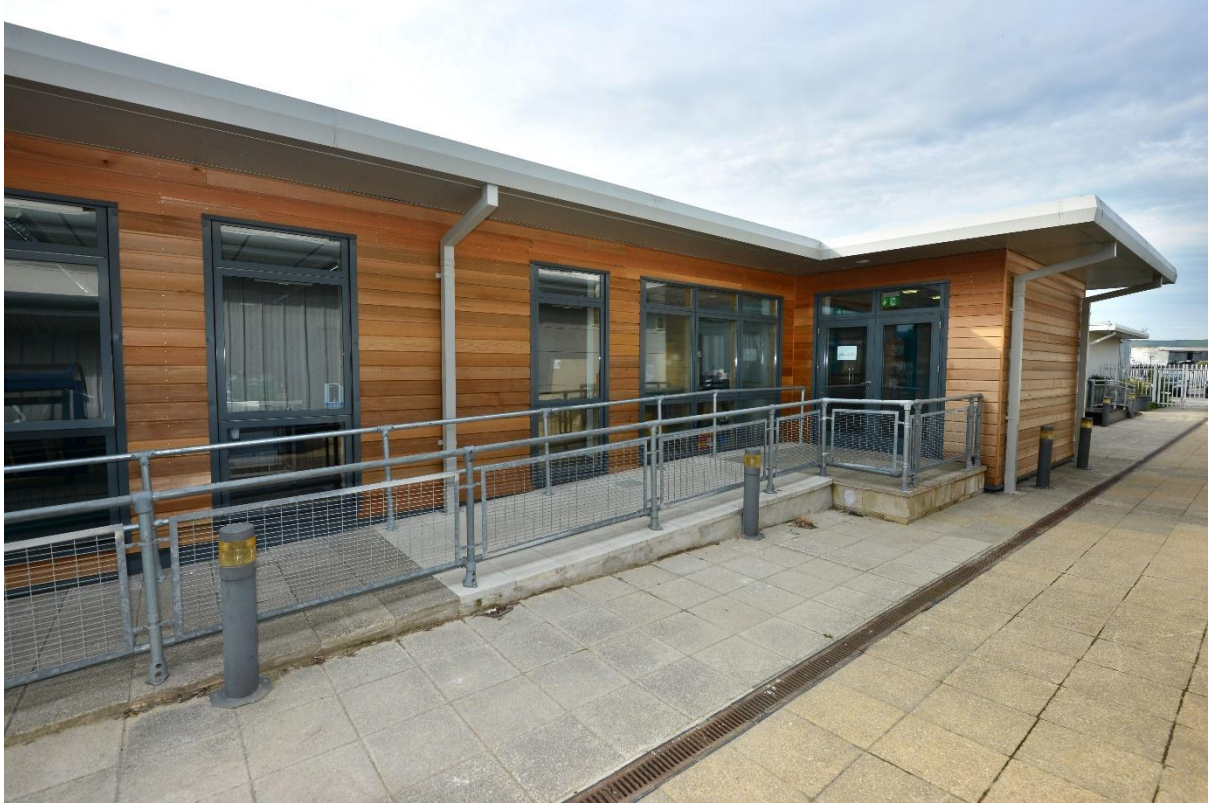
Denton Island Community Centre – Head office Newhaven
