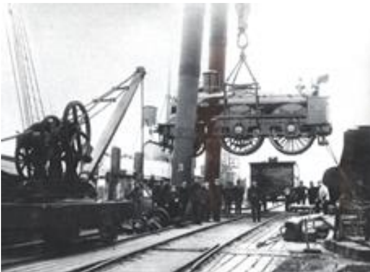
Sheer Legs lifting locomotive bound for France, November 1883. Newhaven Historical Society collection ref: A318-04
