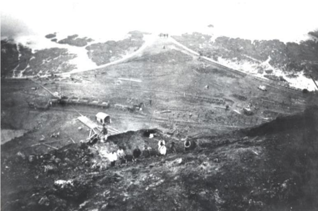
Photo: December 1879 from the cliff top - The breakwater leaves the shore, - notice the men digging away at the cliff for infill. © Newhaven Historical Society A318/322-004
