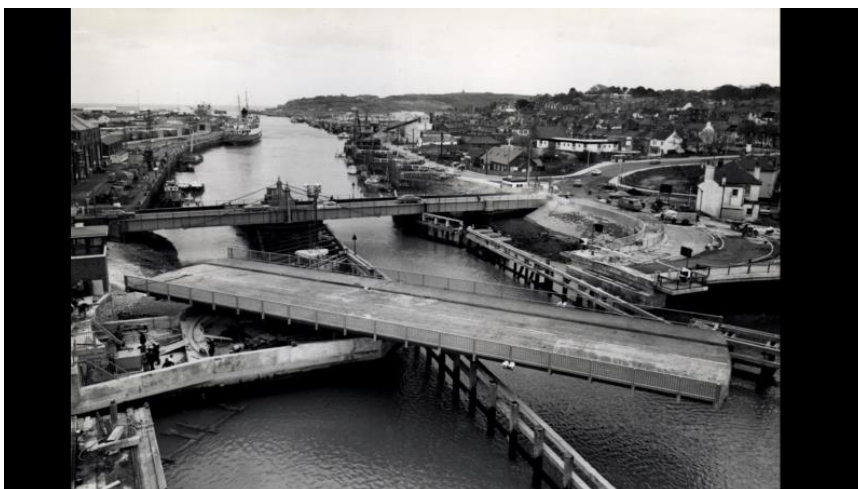
Photo: Testing the New Swing Bridge 1974 - Newhaven Historical Society collection ref: A016-036
