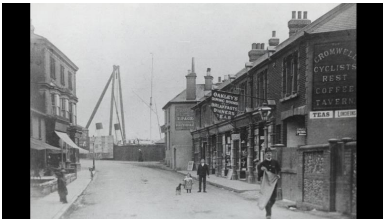
Photo: Bridge street circa 1905 (note: Sheer Legs Crane at the end of the street). Newhaven Historical Society collection ref: A037-034
