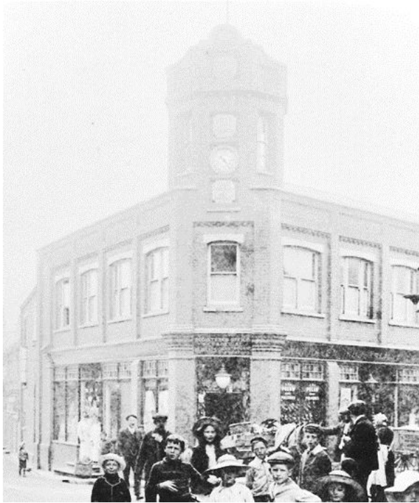
Photo: The Co-op on the corner of Bridge Street and Chapel Street – Newhaven Historical Society collection, ref: A062-072
