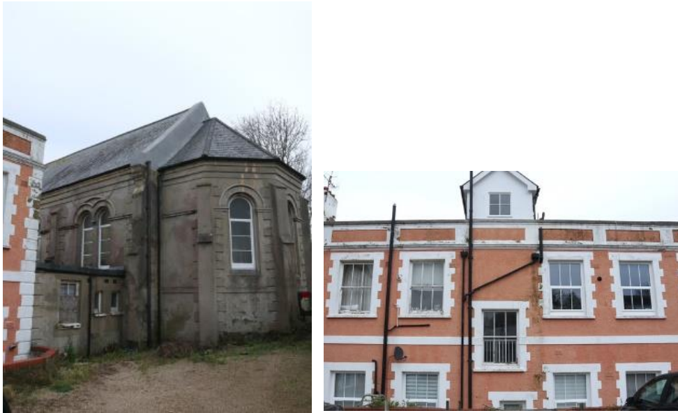
Photos: Convent Buildings- Chapel and Nun's Residences. C Joslin Dec 2023.
